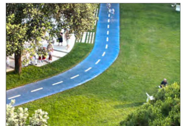
Cycle Path Paving
