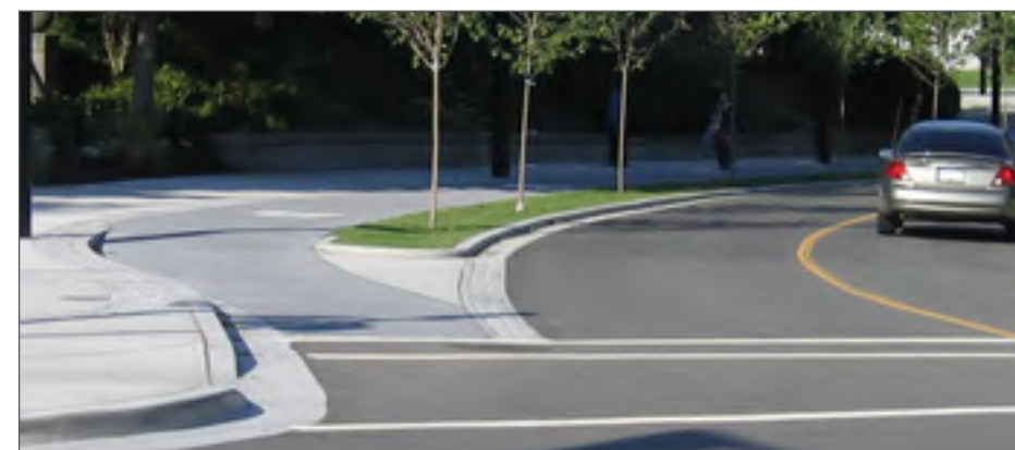
Off-street Bike Lane
